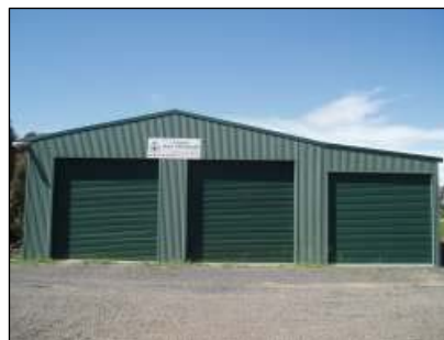
Extensions to the Gundry Rural Bush Fire Brigade shed provide storage for fire fighting vehicles and toilet and washing facilities.
