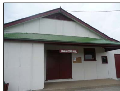
A grant for the Tarago Hall provided an upgrade to the roof, painting and a new rainwater tank was installed.
