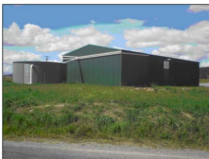
A new toilet and shower block were installed at the Middle Arm Rural Fire Brigade station.
