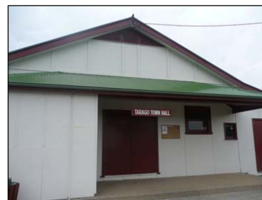
A grant for the Tarago Hall provided an upgrade to the roof, painting and a new rainwater tank was installed.
