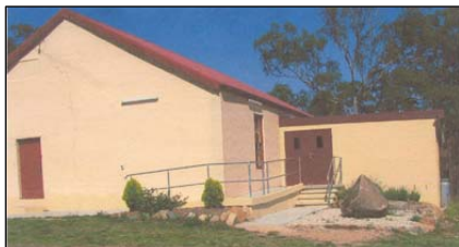
The Bungonia Progress Association completed a new toilet and shower block, disabled access ramp and foyer at the Bungonia Hall.
