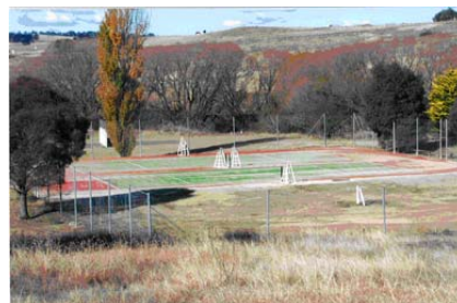
The two new synthetic turf tennis courts at Taralga Tennis Club.
