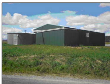
Middle Arm/Mt Wayo Bushfire Brigade improvements to shed
