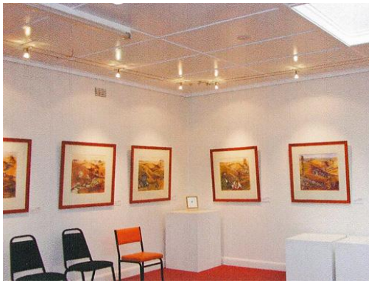
Crookwell & District Art Gallery installation of lighting system in the Gallery
