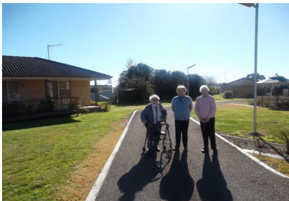
The Legacy Club of Goulburn – Extended existing driveways and installed solar lighting to the area for security and safety
